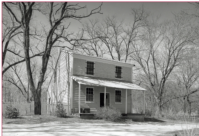
86A-027-11 Coffren Store (NR) 10007 Croom Road Croom
