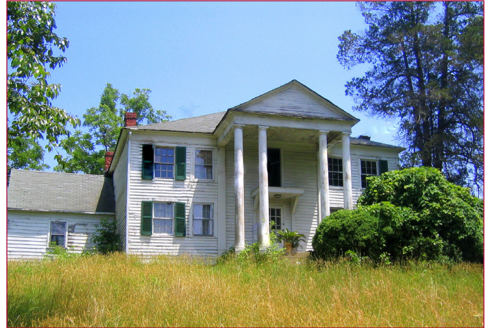
83-009 Dr. William G. Hardy House (Kuehn House/Ellerbrook Farm) 16100 Old Marshall Hall Road Accokeek
