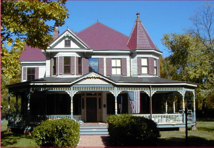
85A-032-09 William W. Early House (NR) 13907 Cherry Tree Crossing Road Brandywine
