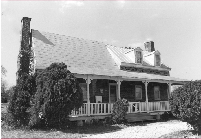
87B-036-16 Grimes House 22609 Aquasco Road Aquasco
