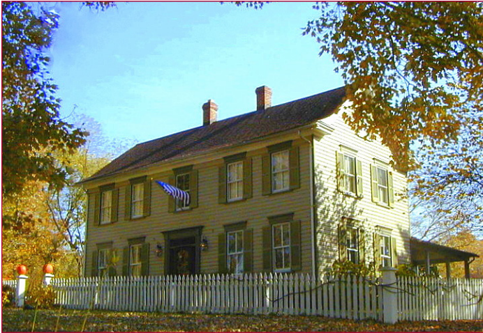
82B-007 William W. Duley House 8100 Croom Road Croom
