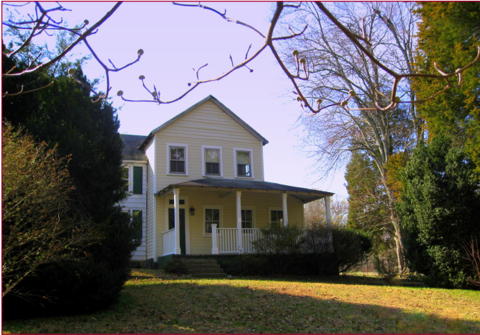
86A-027-24 Croome Settlement School and Croom Institute Site 14409 St. Thomas Church Road Croom
