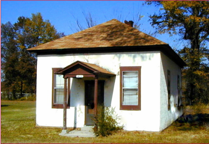
85A-032-30 Old Bank of Brandywine 14110 Brandywine Road Brandywine
