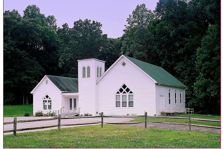
86B-005 Nottingham-Myers Methodist Church 15601 Brooks Church Road Croom
