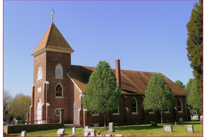
84-023-10 St. Mary's Roman Catholic Church and Cemetery 13407 Piscataway Road Piscataway
